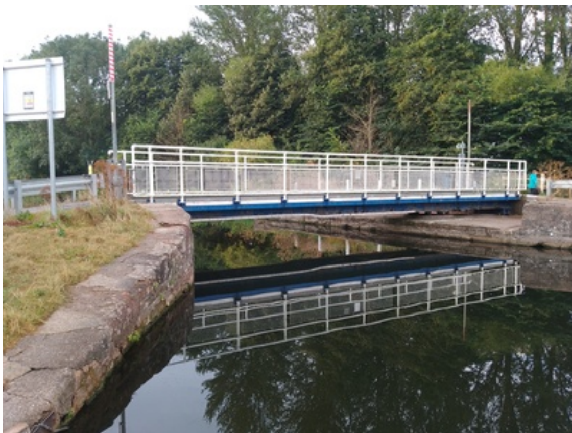
Bridge on Clapperbrook Lane
