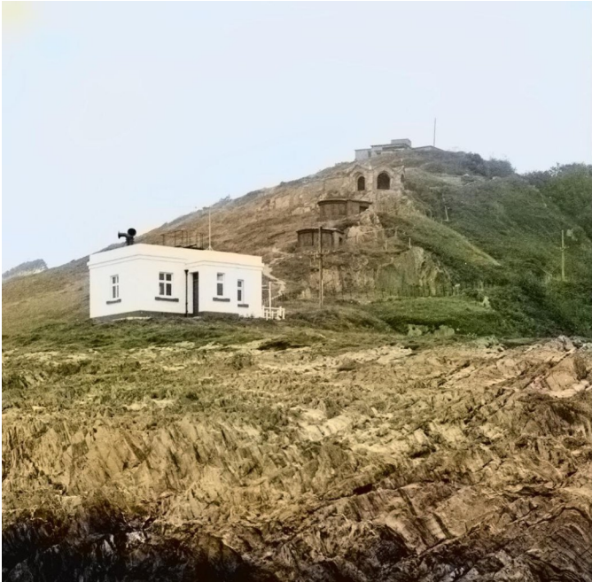
Fog Station Machinery and Control Building
