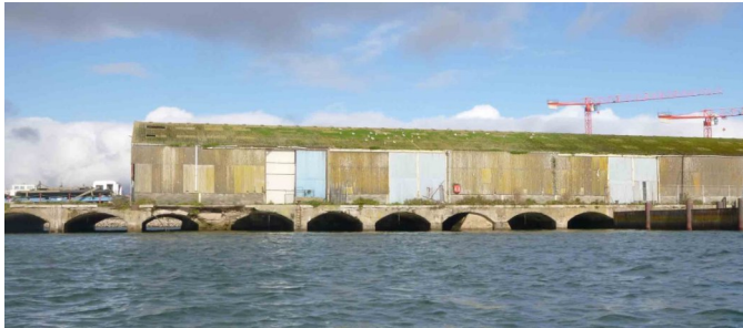
Trinity Pier Just Before the Warehouses Were Demolished
