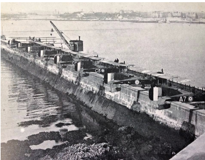
Seaplanes Parked on the Breakwater
