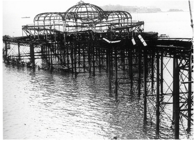
The Wrecked Remains of the Pier
