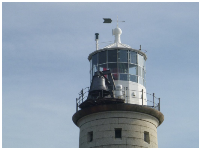
The Lighthouse Lantern and Fog Bell
