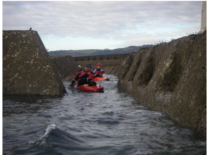
Concrete Wavebreaker Blocks (Left)
