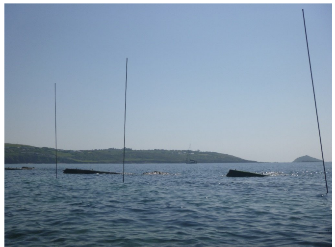
Newly Laid Blocks with Orientation Poles Intact
