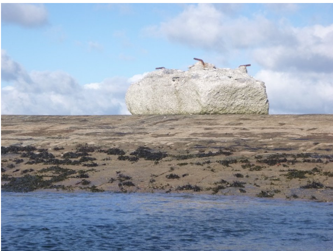
100t Block on top of the Breakwater
