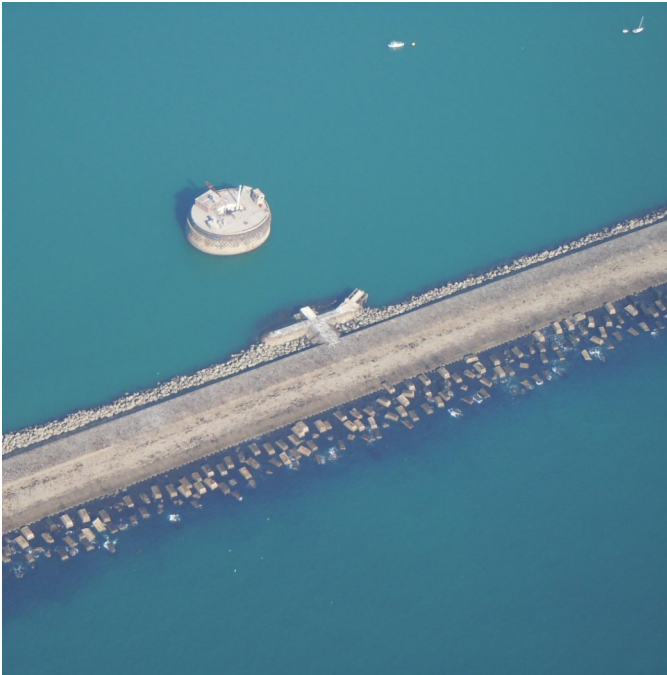
Aerial View of Wavebreaker Blocks (Stephen Johnson)
