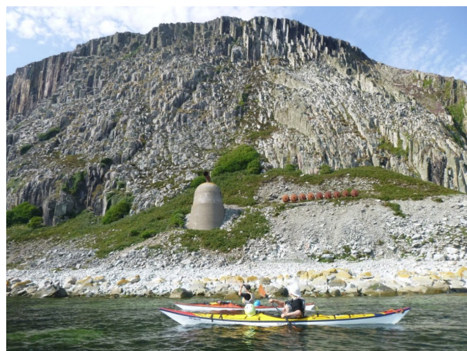
Disused Fog Station
