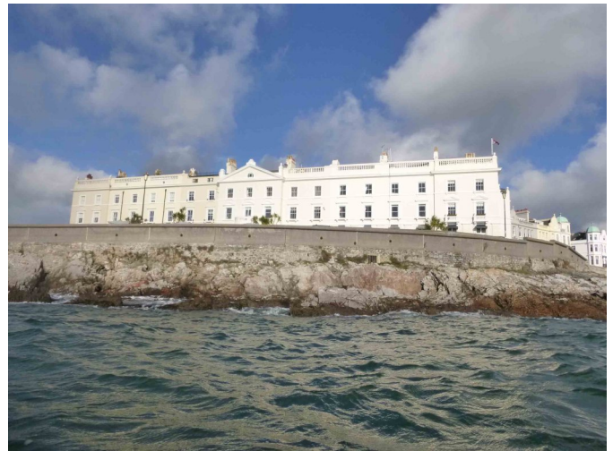
West Hoe Terrace
